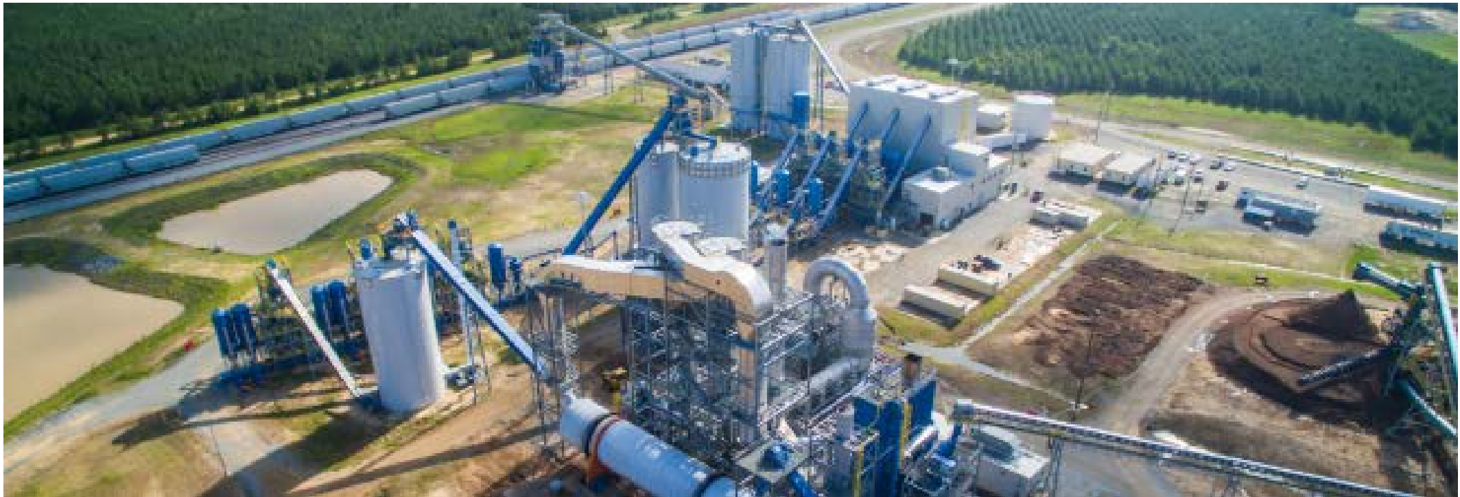
Drax Biomass 450,000 ton per year pellet fuel production plant.
