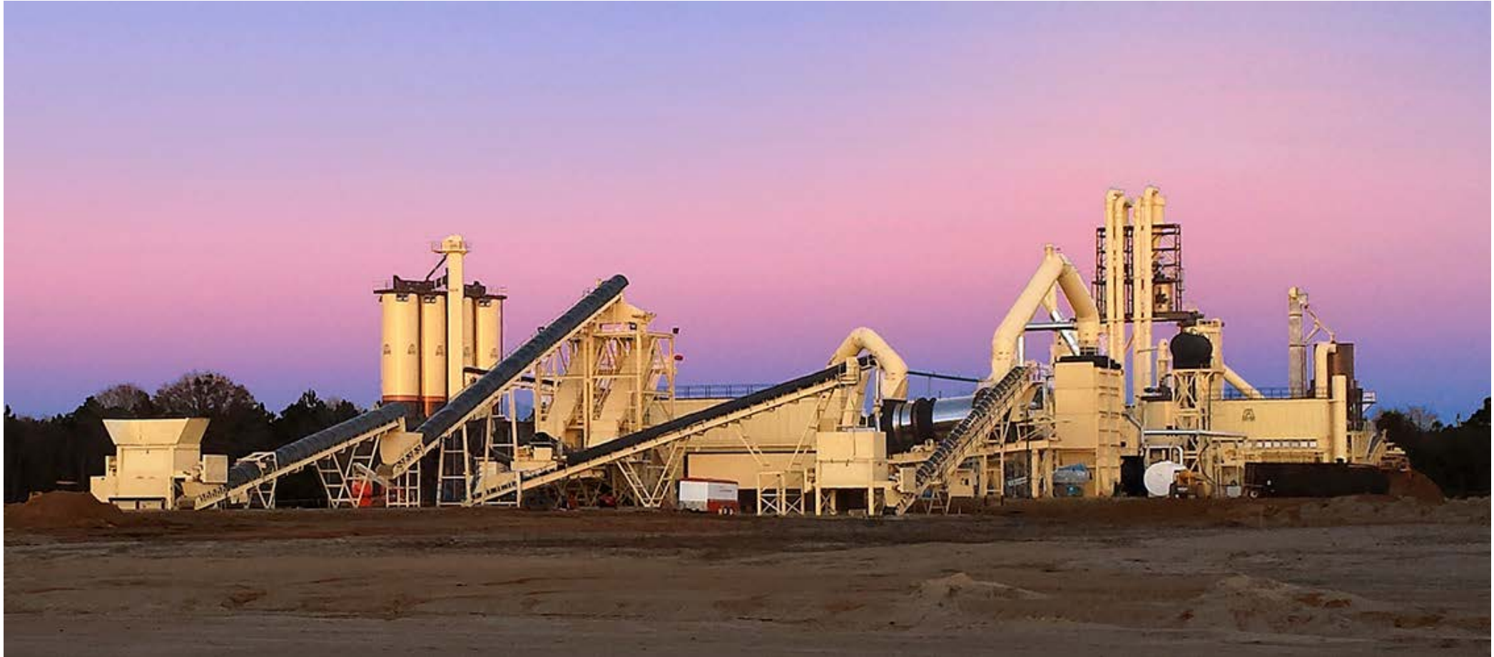
Photo of Fram Renewable Fuels 475,000 ton per year plant in Hazelhurst GA, built by Astec Industries
